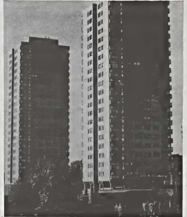
High-rise blocks: Badly-designed and sloppily built
